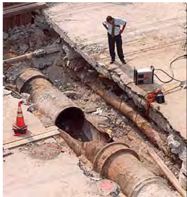
Figure 3. An official surveys the gaping hole and broken 40-in. water main at Howard and Lombard streets (see Reference 10).
